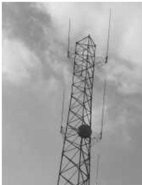
Shown here is a photo of the Centre County EMA tower on Rattlesnake Mountain which is home to PARA's .43 Repeater. This photo shows the antenna that failed and is in the process of being replaced.
