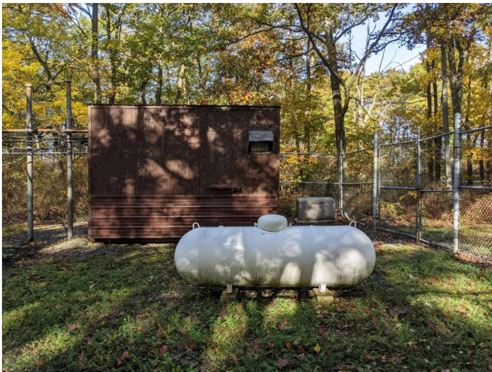
Repeater shed, generator, and propane tank
